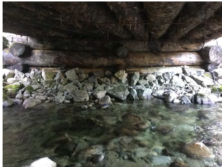
Left Bank Abutment when facing downstream
