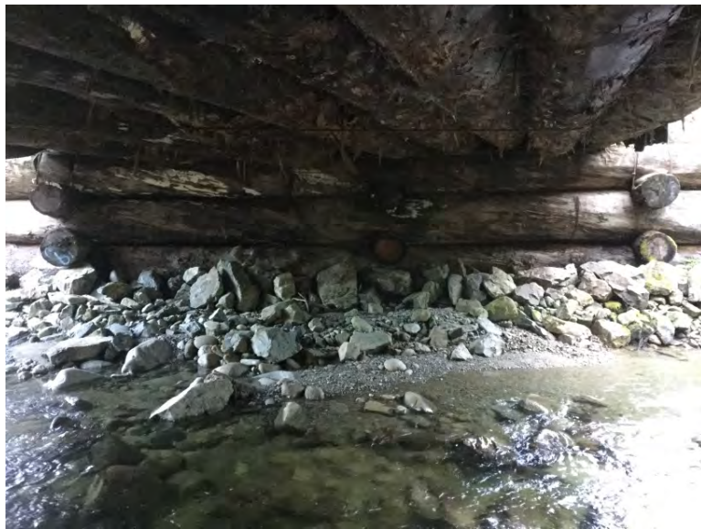
Right Bank Abutment when facing downstream
